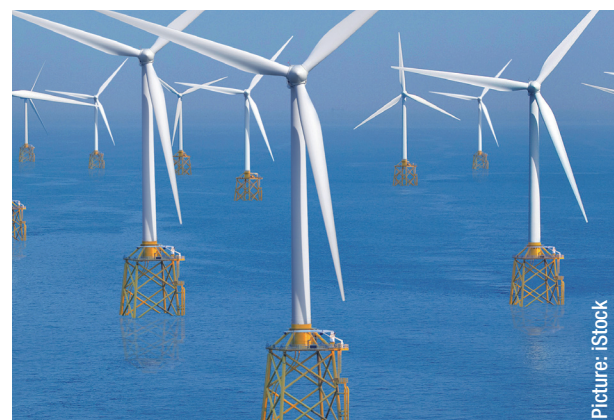
Jackets for Offshore-Windparks
